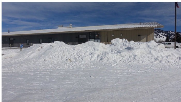
Fire&EMS/Fair Office, West side
