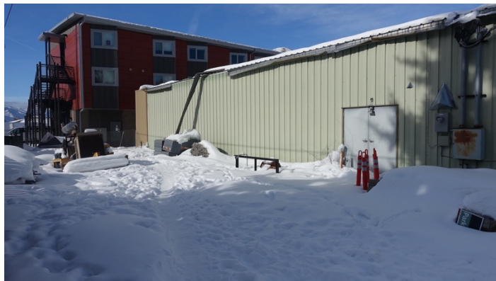
Fair Building, South side
