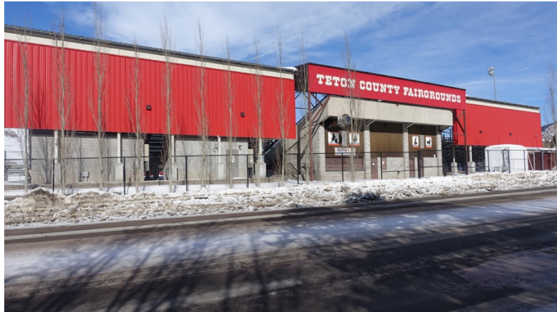
South Elevation, Rodeo Arena Covered Grandstands
