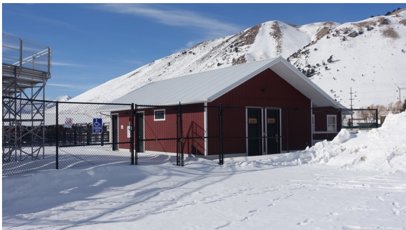
East side, Bathrooms
