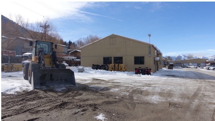
Public Works Shop, East side
