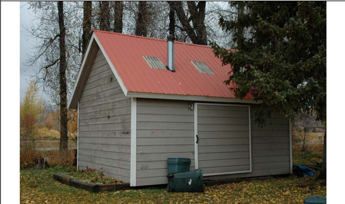
Photograph 10 East and south elevations of shed, camera facing northwest. (photographed October 2016)
