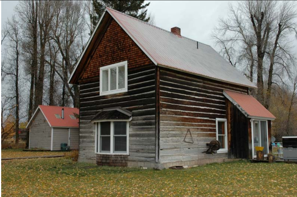
Photograph 5 South and east elevations of house, camera facing northwest. (photographed October 2016)
