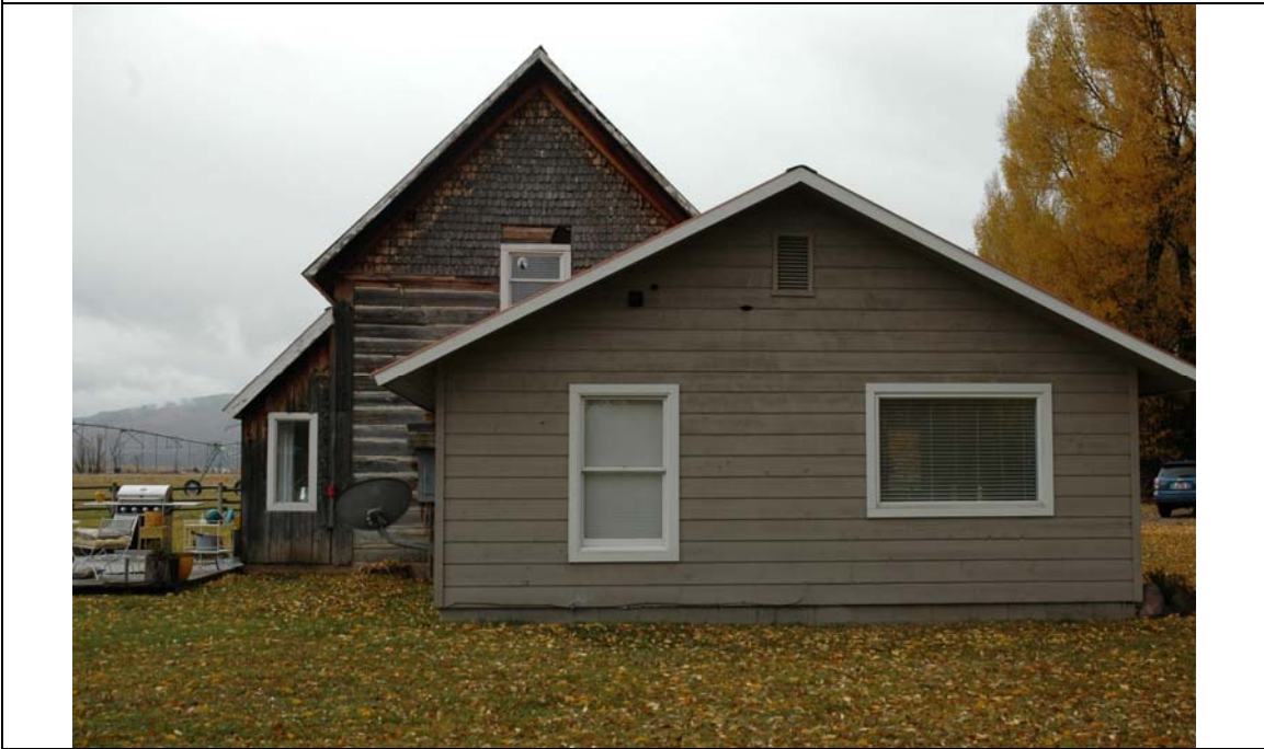
Photograph 8 North elevations of house and addition, camera facing south. (photographed October 2016)
