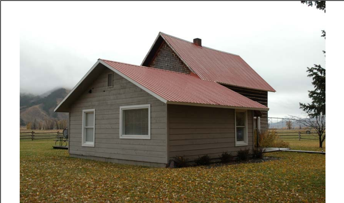
Photograph 9 North and west elevations of addition, camera facing southeast. (photographed October 2016)
