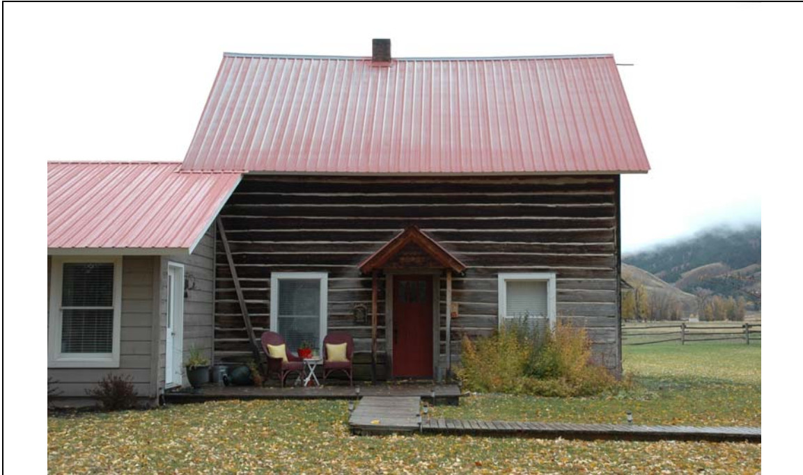
Photograph 1 West elevation of house, camera facing east. (photographed October 2016)
