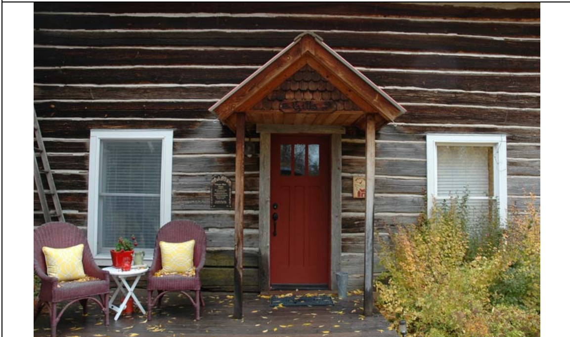
Photograph 2 West elevation of house, façade detail, camera facing east. (photographed October 2016)
