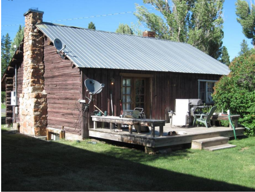
First Baptist Church of Jackson Hole Parsonage, South Elevation, Longfield, 2009
