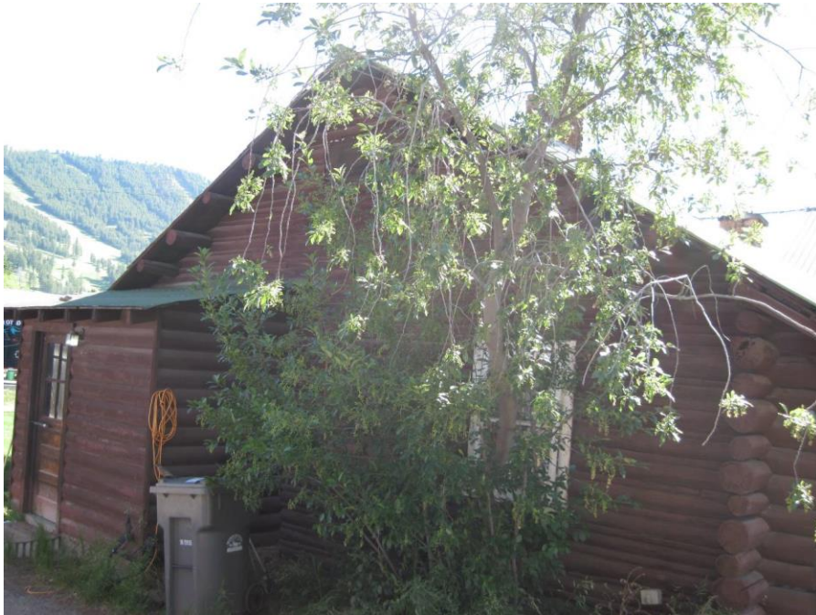
First Baptist Church of Jackson Hole Parsonage, East Elevation, Longfield, 2009
