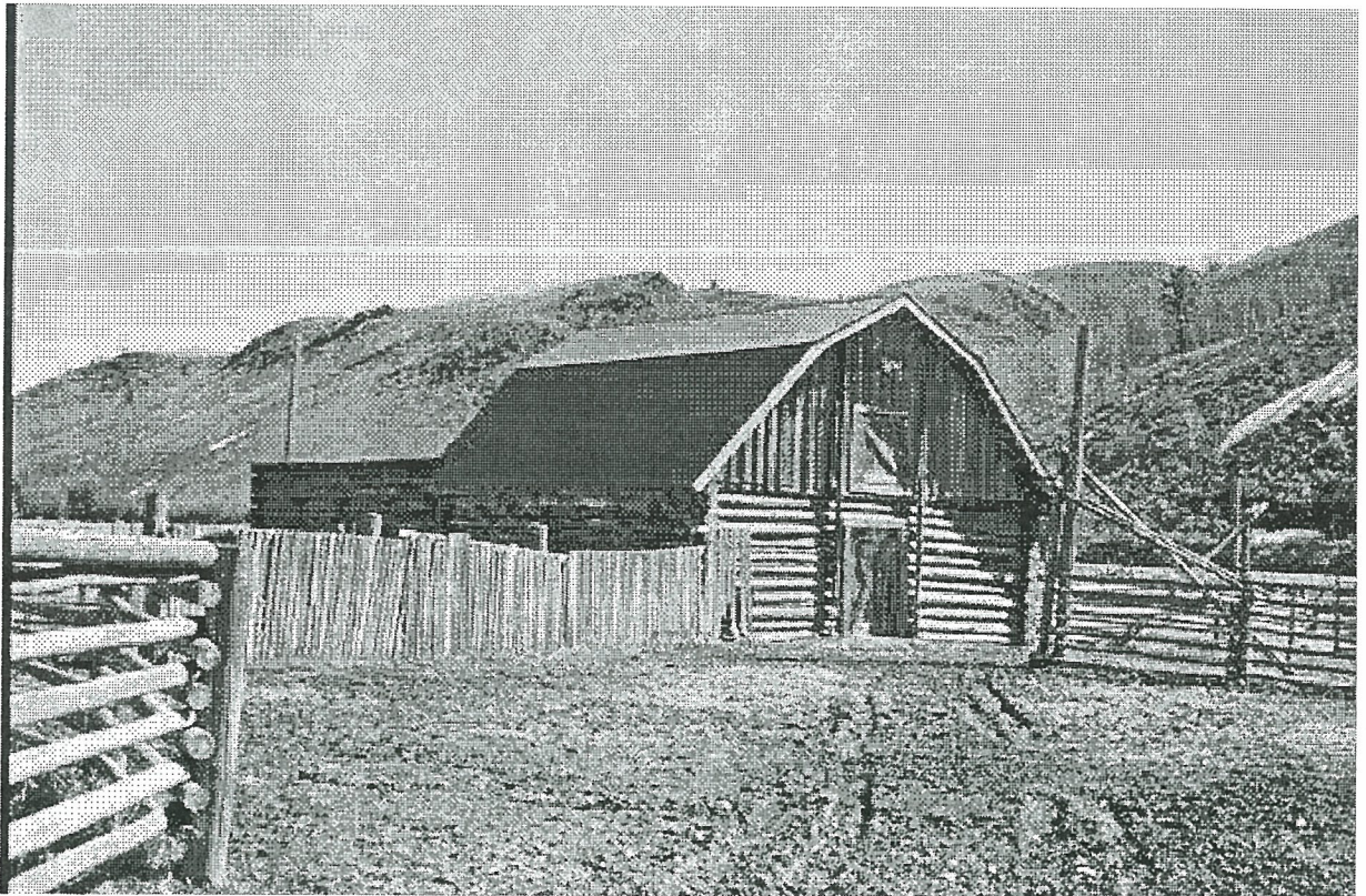
Feature 9. Log barn. South and west elevations.
