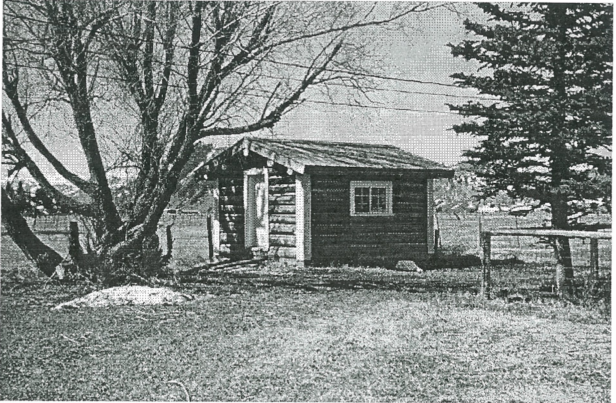
Feature 11. Single-cell house. East and north elevations.
