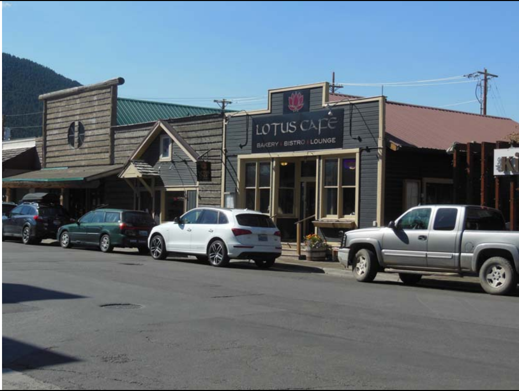
Photograph 3 North and west elevations of complex, camera facing southwest.
