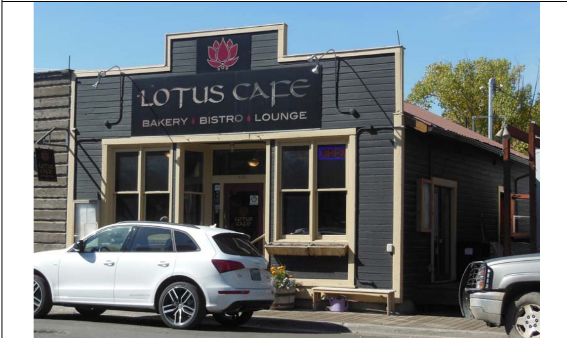
Photograph 2 East and north elevations of shop, camera facing southwest. (photographed October 2016)
