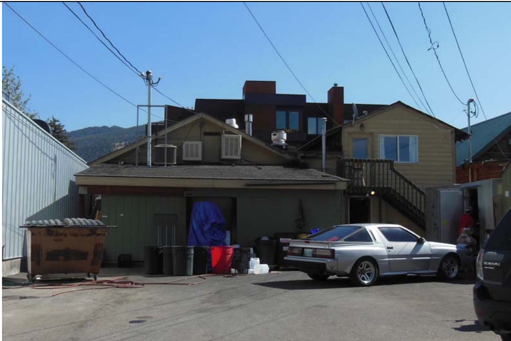
Photograph 4 East elevation of complex, camera facing east.
