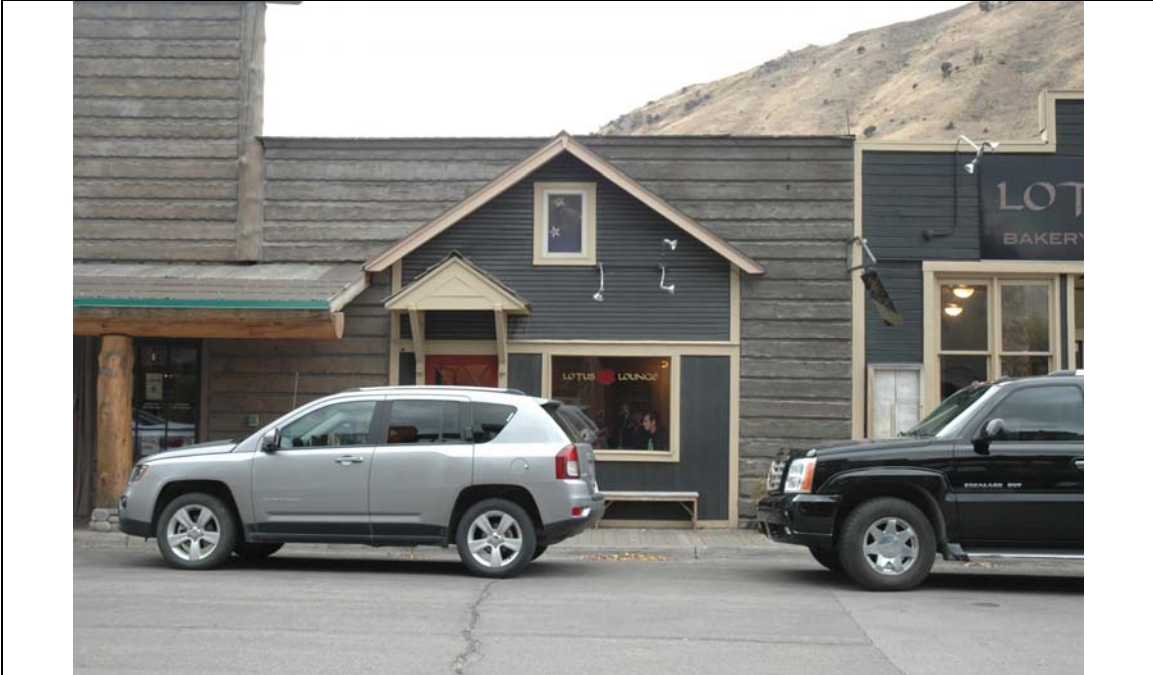
Photograph 5 West elevation of south half of complex, camera facing west.
