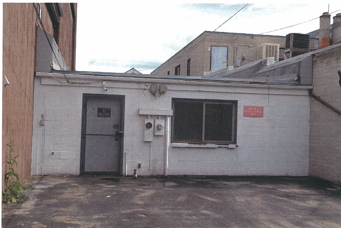
Frontier Saloon / Boyer's Rod and Reel / Indian Arts and Crafts, south elevation, looking north. Photo: Michael Cassity, 2005.
