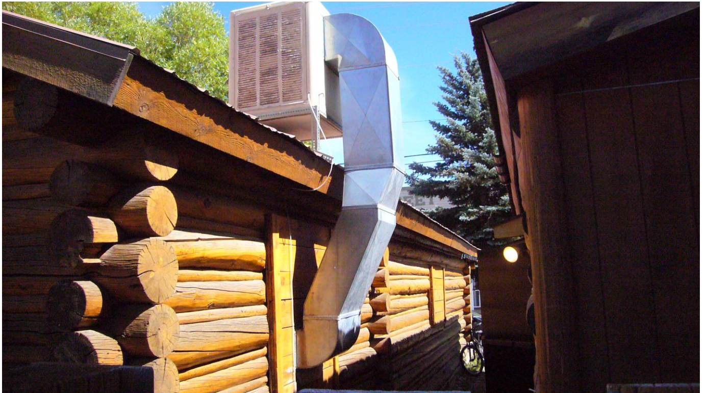
Ellen Walker Smart Shoppe, South Elevation, Longfield, 2009
