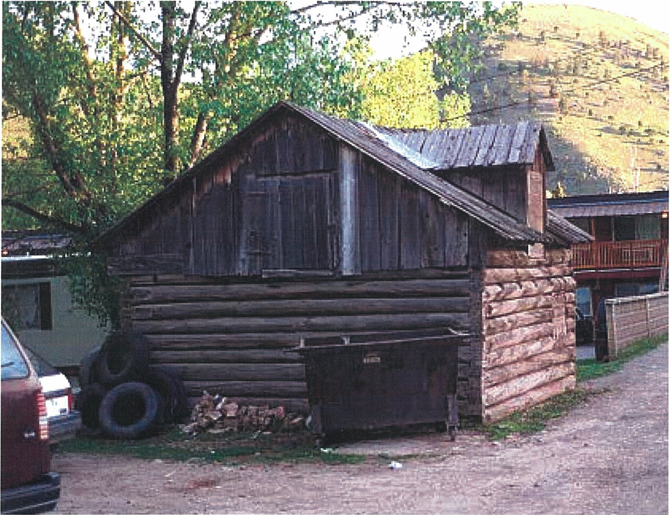
Elias Wilson Barn, Jackson, Wyoming. South and east elevations, looking north. Photo: Michael Cassity, 1999.
