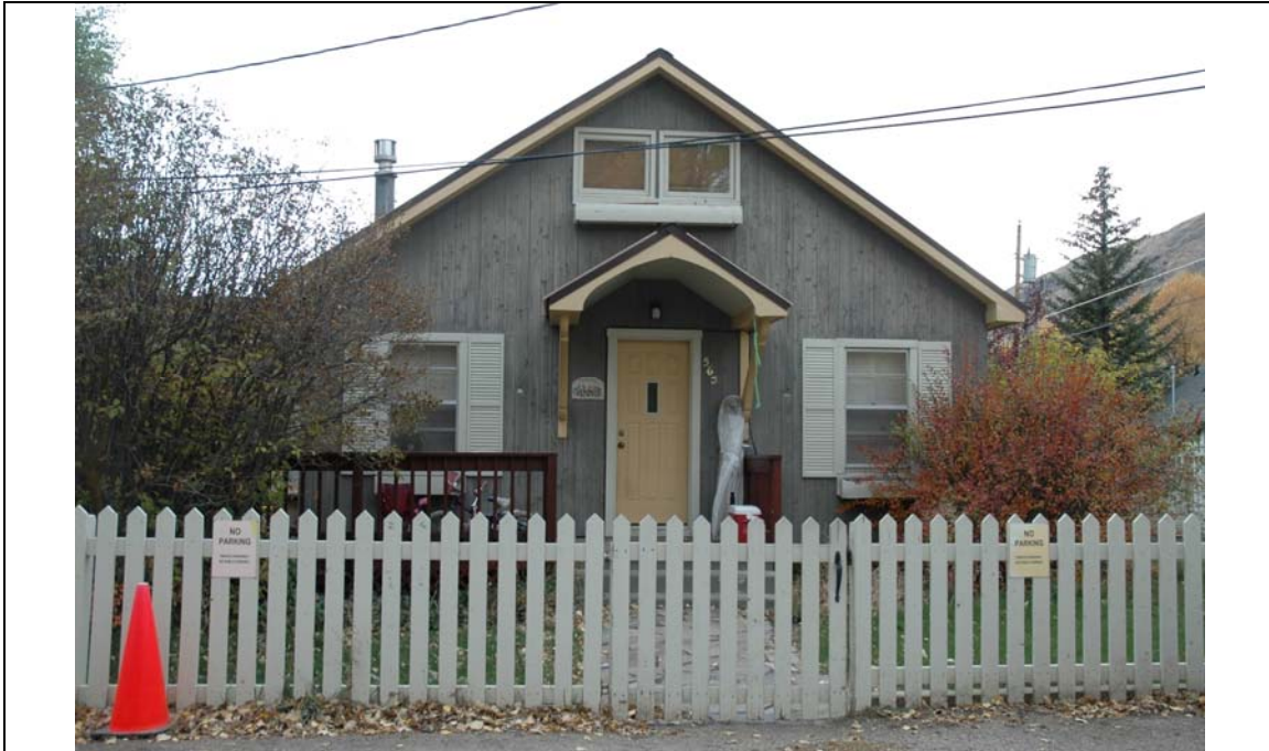
Photograph 1 East elevation of house, camera facing west. (photographed October 2016)
