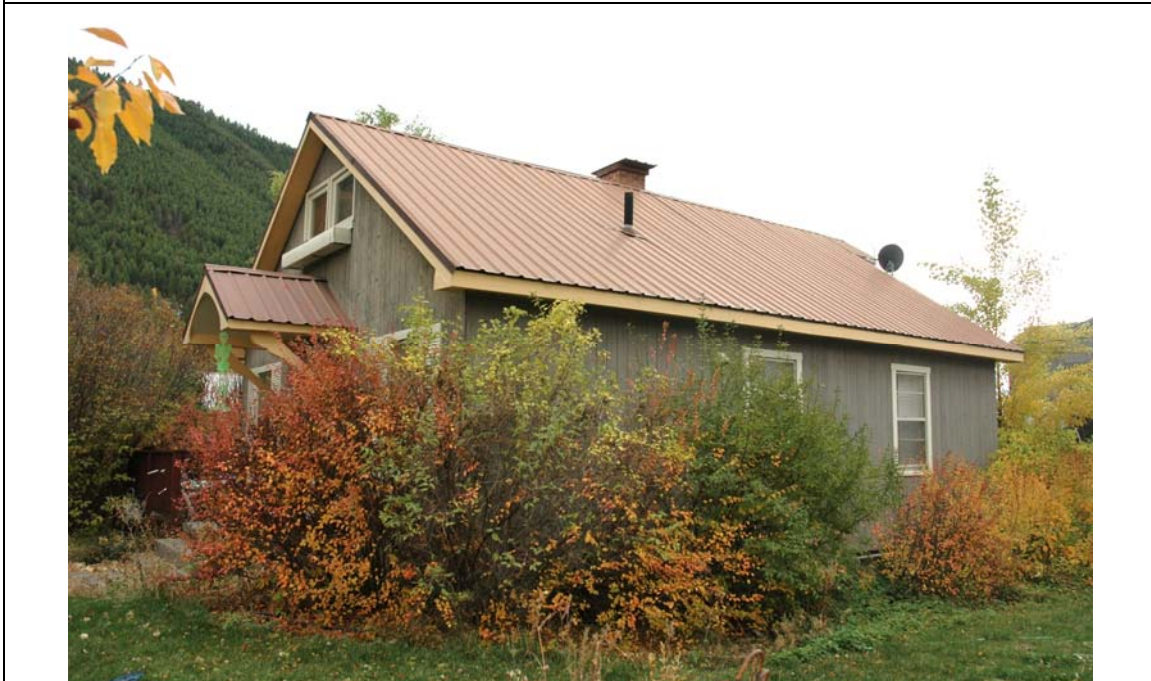
Photograph 2 East and north elevations of house, camera facing southwest. (photographed October 2016)
