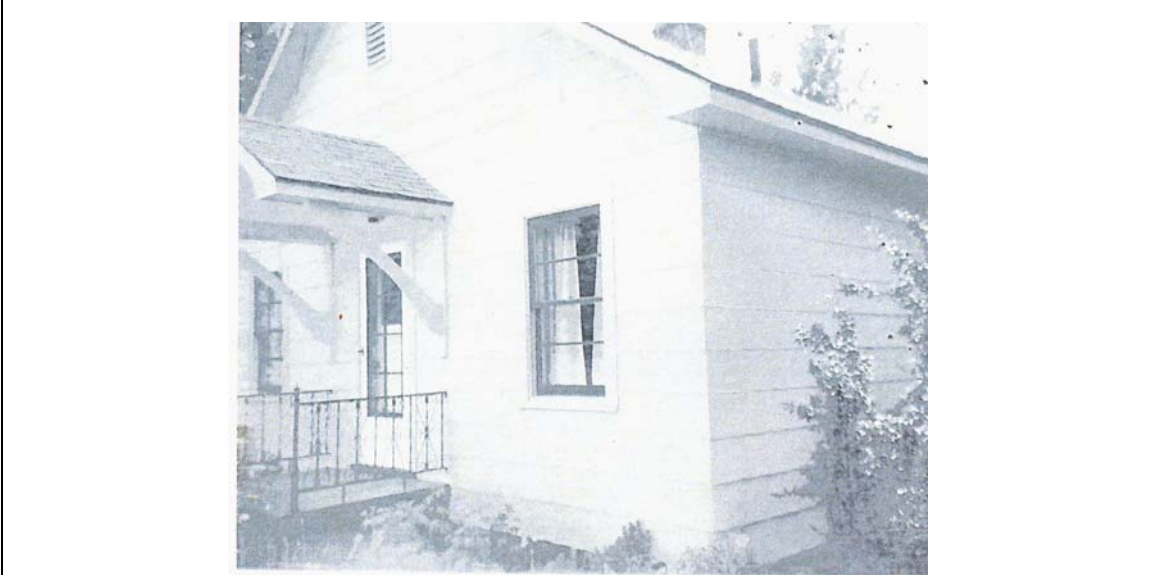
Clissold House , east and north elevations, circa 1960. (courtesy Teton County Assessor's Office)
