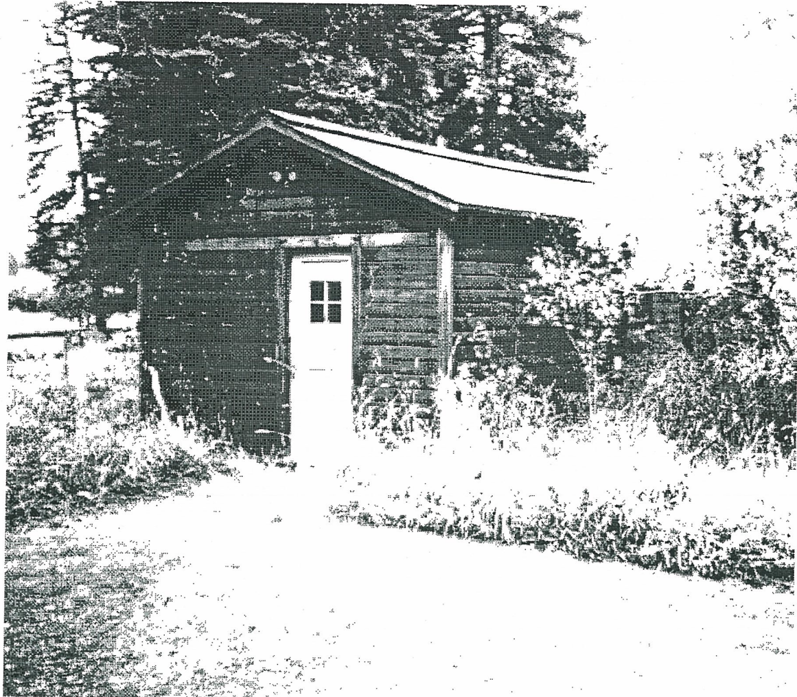
Feature 2. Well house / Pump house.
