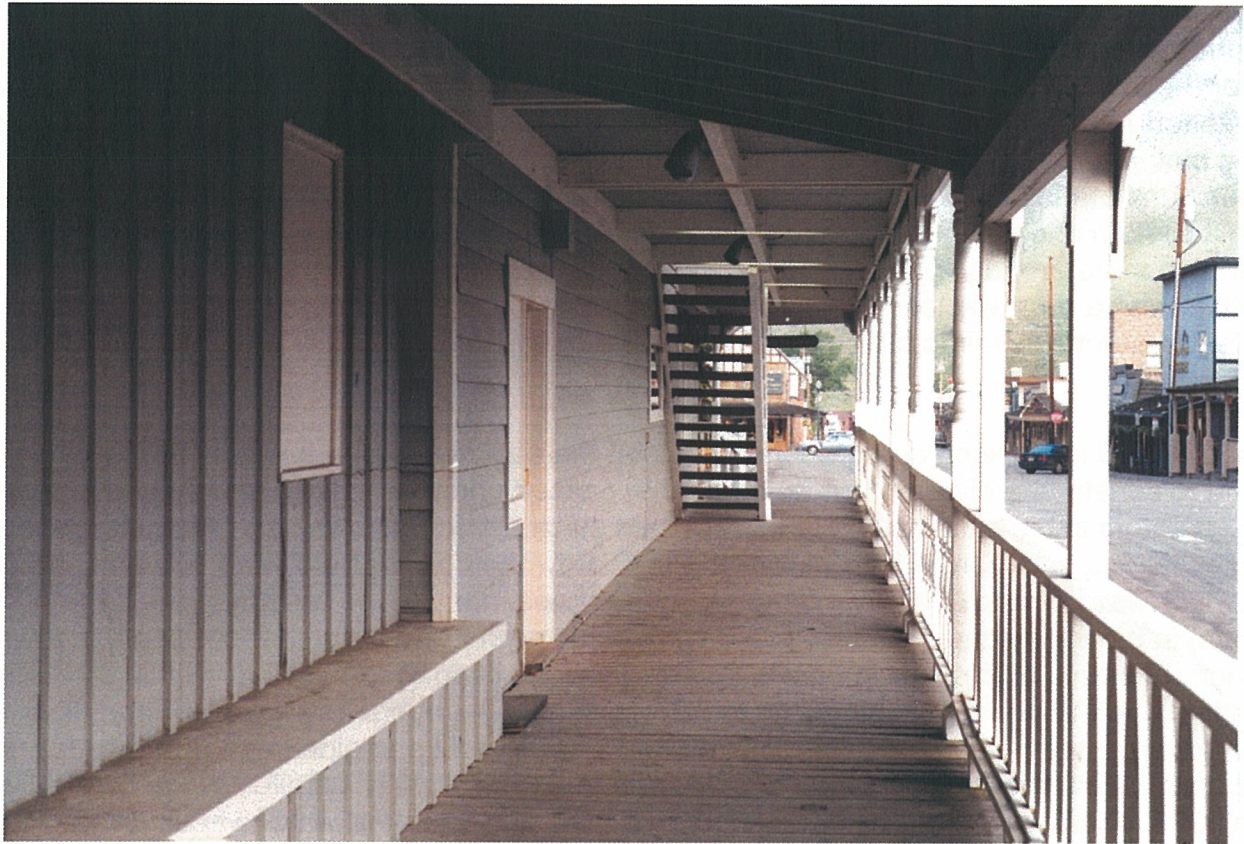
Benson Building, north elevation, ground level, looking west. Note stairway in original location and also the inset in the elevation and the sloping canopy in the foreground where the building was extended to the east. Photo: Michael Cassity, 1999.
