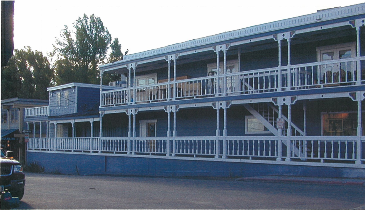
Benson Building / Jackson Hole Light and Power Company Building, north elevation. Photo: Michael Cassity, 2004.
