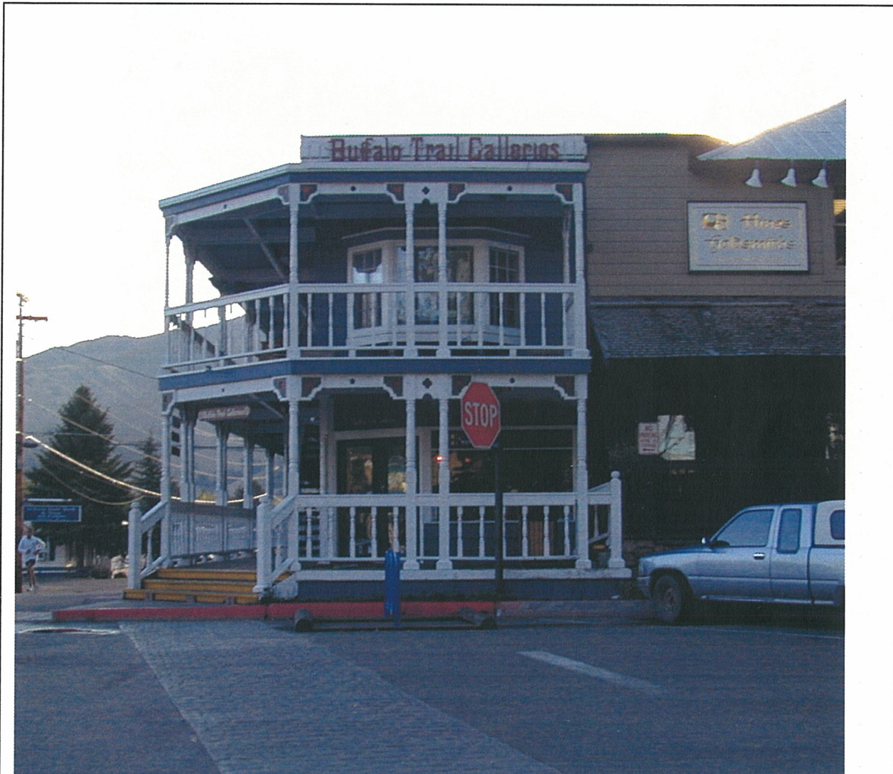
Jackson Hole Light & Power Building / Benson Building. West elevation. Originally, the elevation extended south to the north elevation of the Clubhouse at a point directly below the eave of the hipped roof visible in the upper right. Photo: Michael Cassity, 2004.
