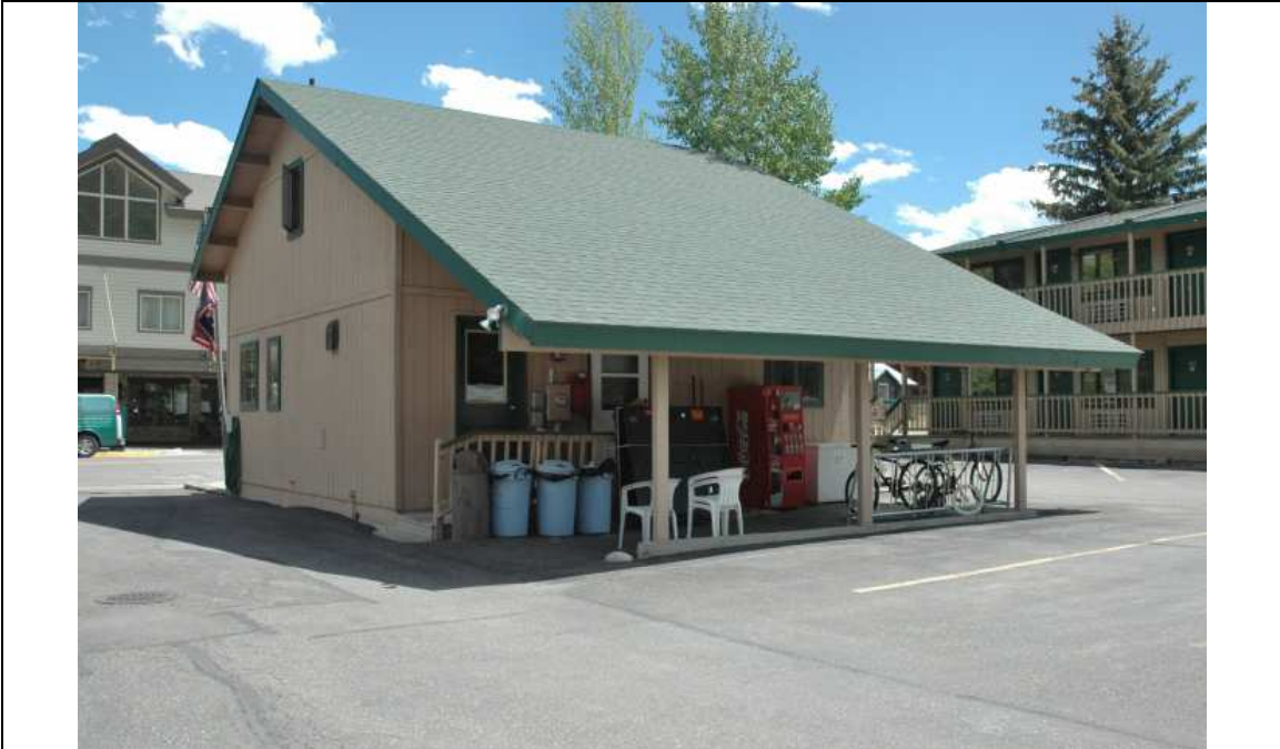
Photograph 8 Anglers Inn, north and west elevation of office (1987, non-contributing), camera facing southeast. (photographed June 2, 2013)
