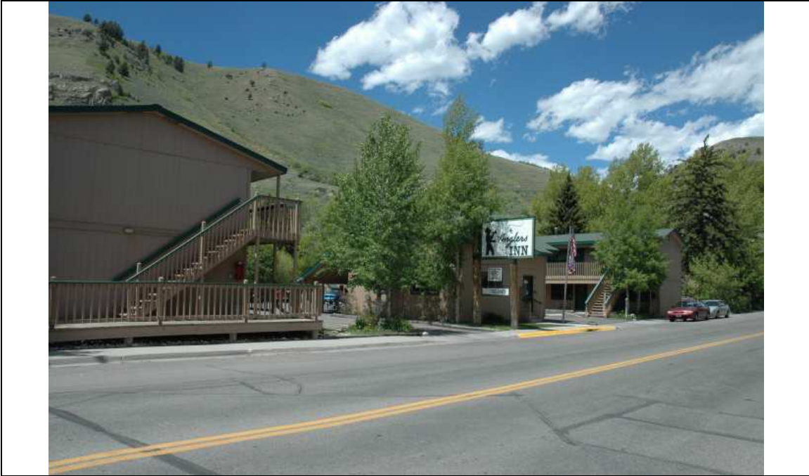
Photograph 1 Anglers Inn, view of site (1934-1987, non-contributing), camera facing northwest. (photographed June 2, 2013)
