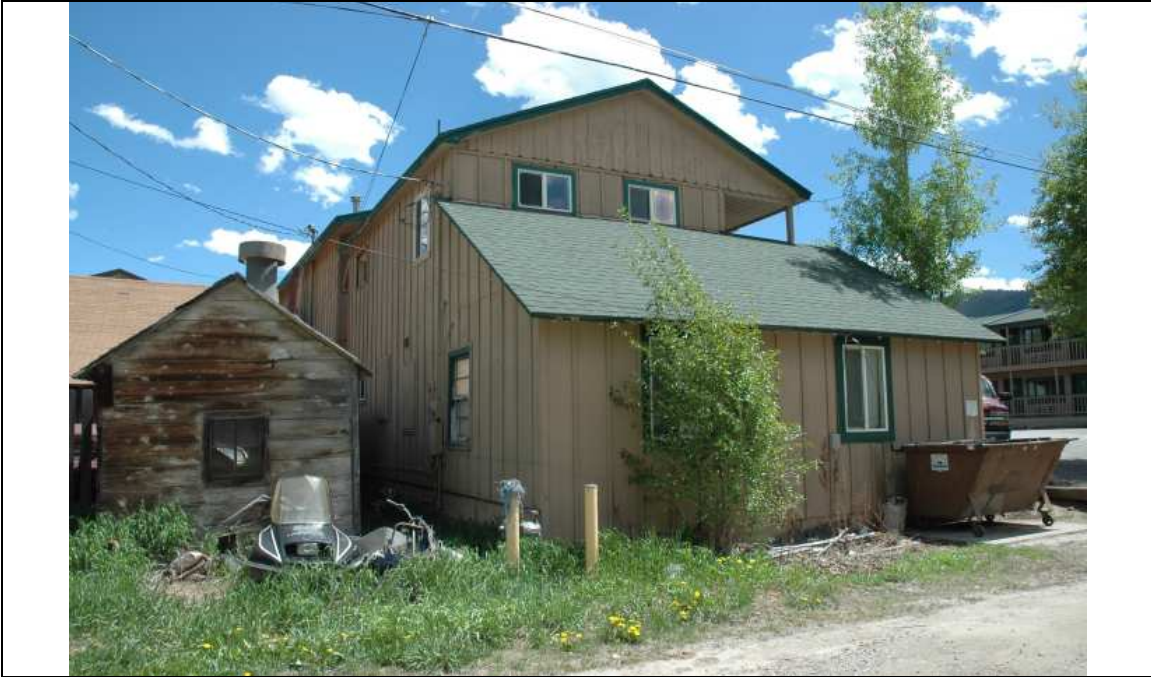
Photograph 3 Anglers Inn, north and west elevations (circa 1934, non-contributing), camera facing southeast. (photographed June 2, 2013)
