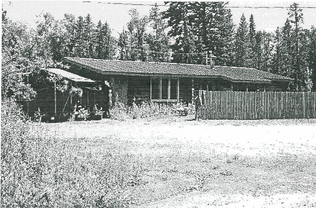
Feature 8. Bunkhouse. North and west elevations.
