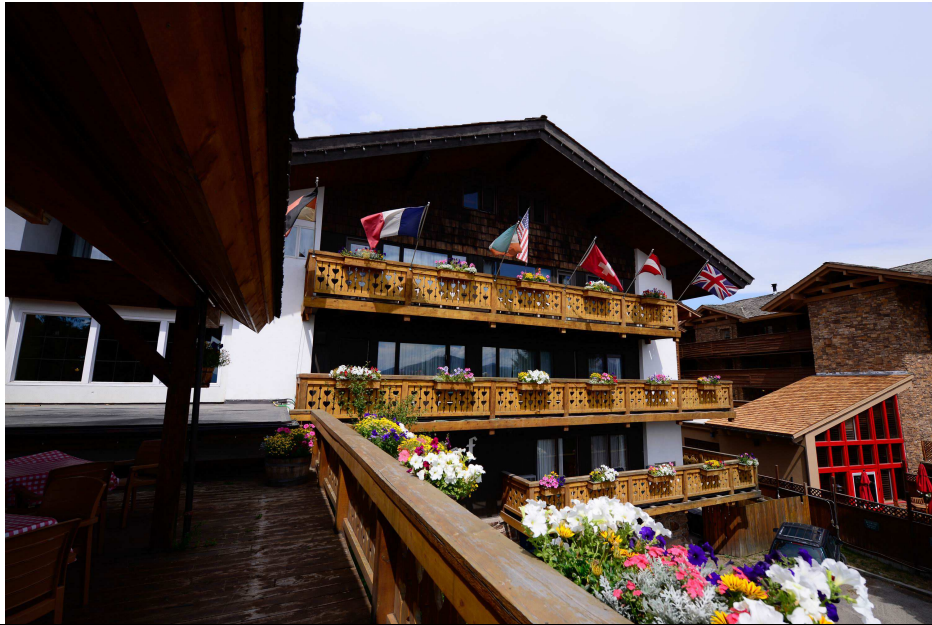
Photograph 5 Alpenhof Lodge, south elevation balconies, camera facing northeast. (photographed August 21, 2013 by Brian Herbel)
