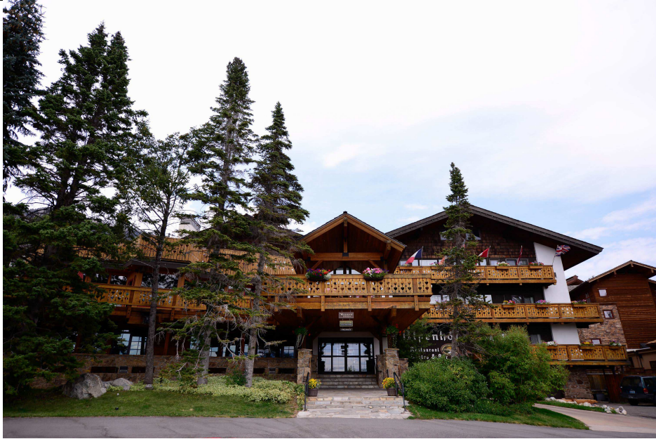
Photograph 1 Alpenhof Lodge, south elevation, camera facing north. (photographed August 21, 2013 by Brian Herbel)
