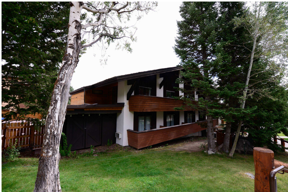
Photograph 6 Alpenhof Lodge, west elevation, camera facing southeast. (photographed August 21, 2013 by Brian Herbel)
