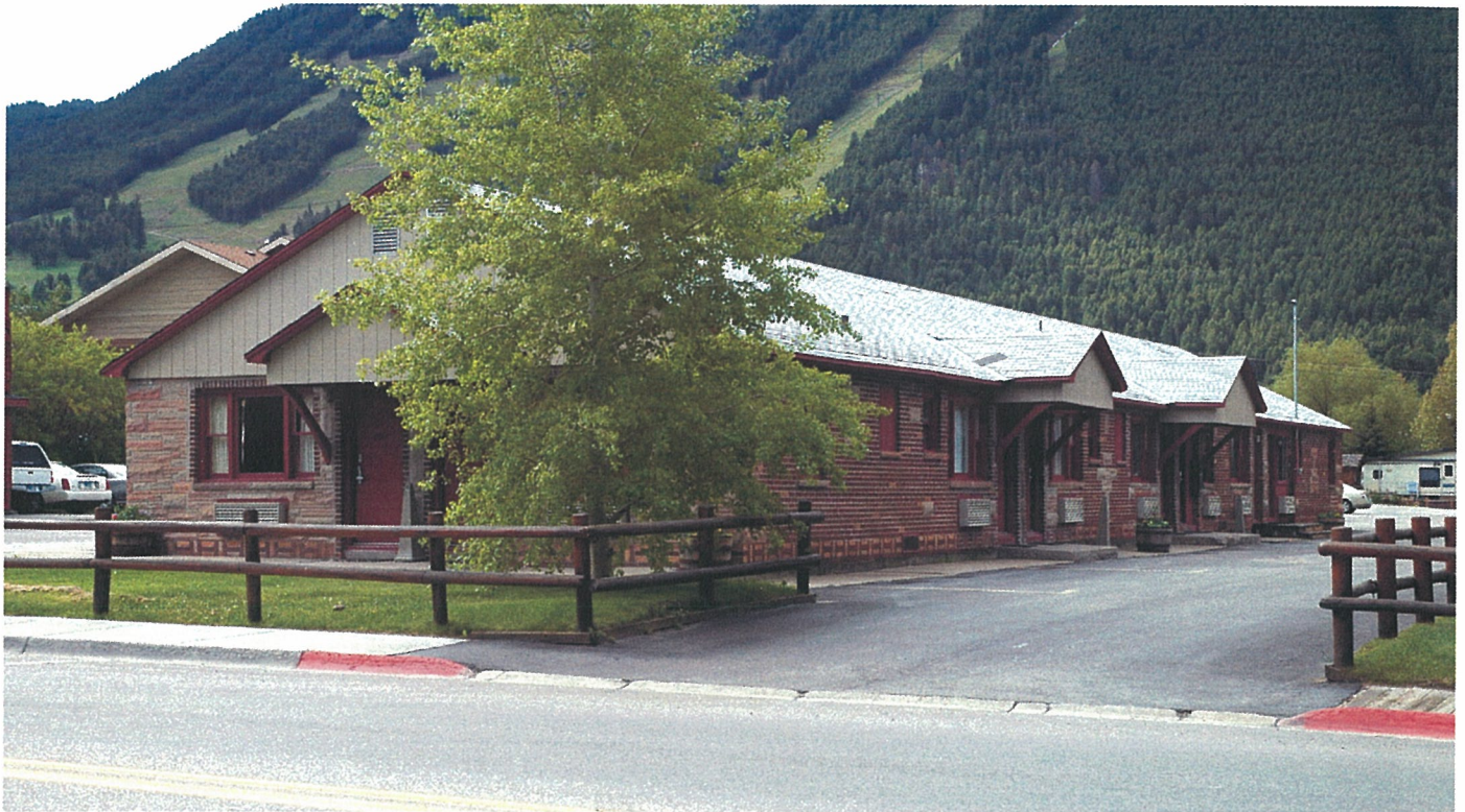
6 – K Motel, Jackson, Wyoming. Remaining building, looking southeast. Photo: Michael Cassity, 2005.
